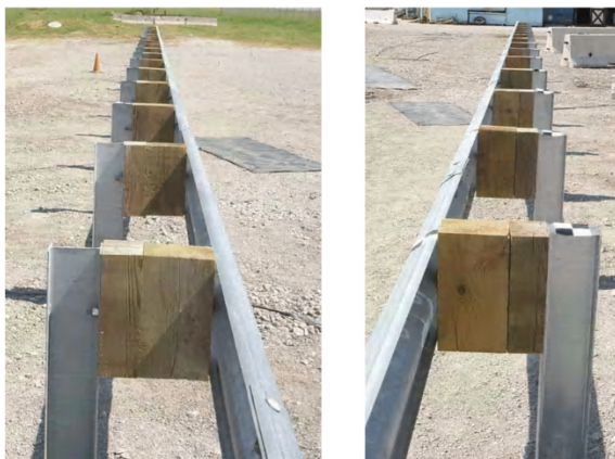
Рис. 4. Система Midwest Guardrail System (MGS)
